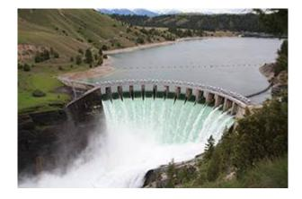
In comparison to water, capacitor is like a dam in the middle of our water flow, storing water for some time. In both cases, if no current/water flows into or out of the capacitor/dam, the water level/voltage remains constant. And the more current/water flows in or out, the faster the water level/voltage changes.
